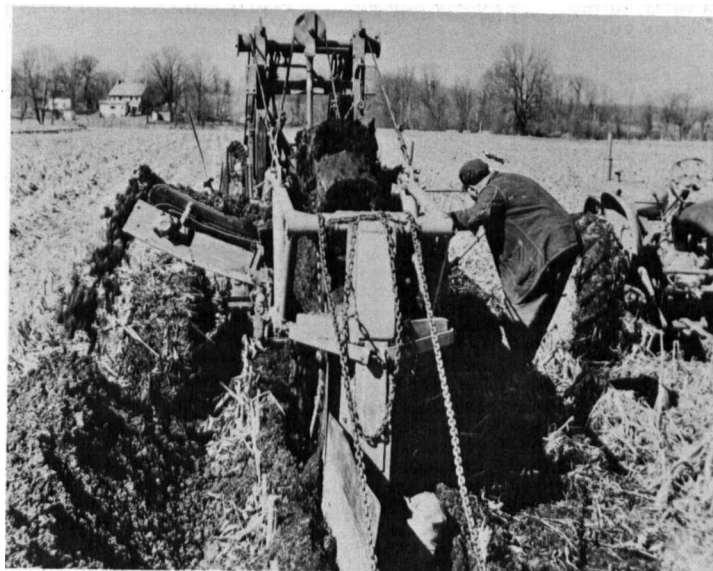
Figure 3.—Installing tile in Luray silty clay loam to provide the necessary drainage for farming.
