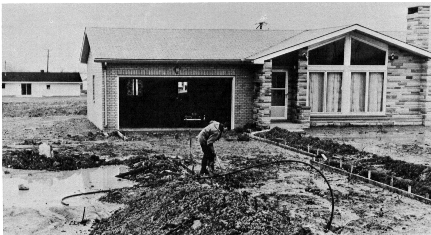
Figure 4.—Removal of surface water is needed on the moderately well drained but slowly permeable Rittman soils if they are used for housing.
